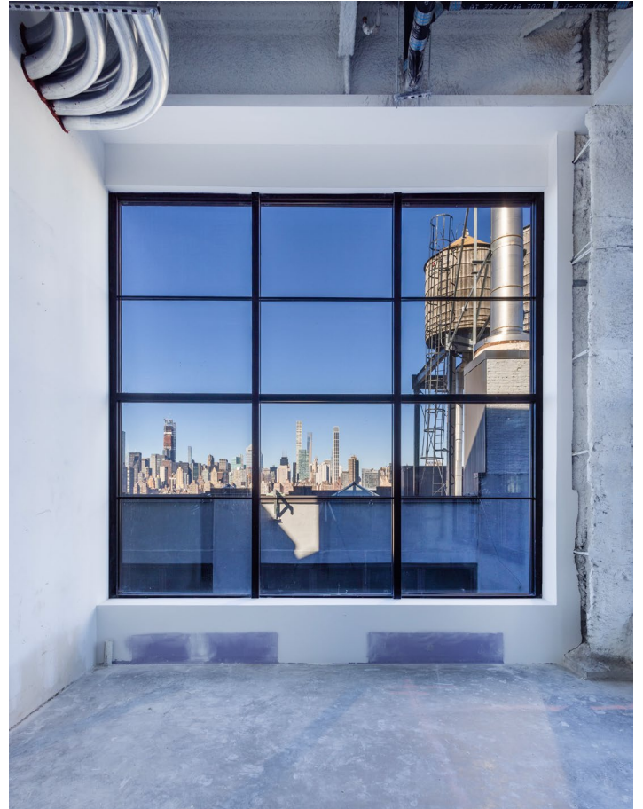
Oversized SAFTI FIRST fire rated fixed unit Installed by Skyline Windows
